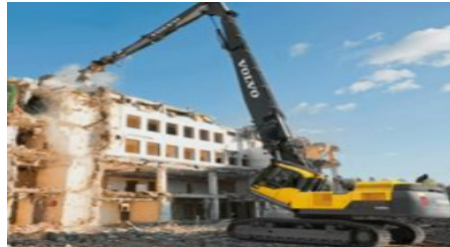
ढहाना (TO DEMOLISH)
