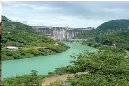
Bhakra Nangal dam
