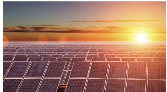
Solar power plant
