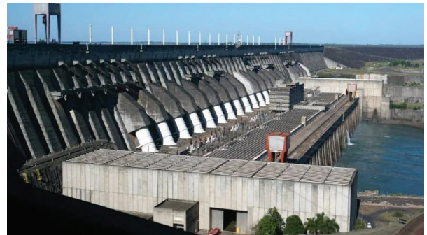
Hydro electric power plant
