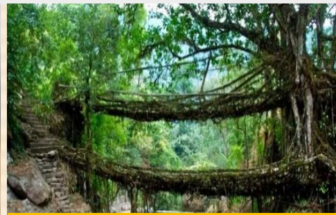
Tree Root Bridges The Tree Root Bridges of Cherapunji are made up of Roots of Living Trees that resemble a suspension bridge
